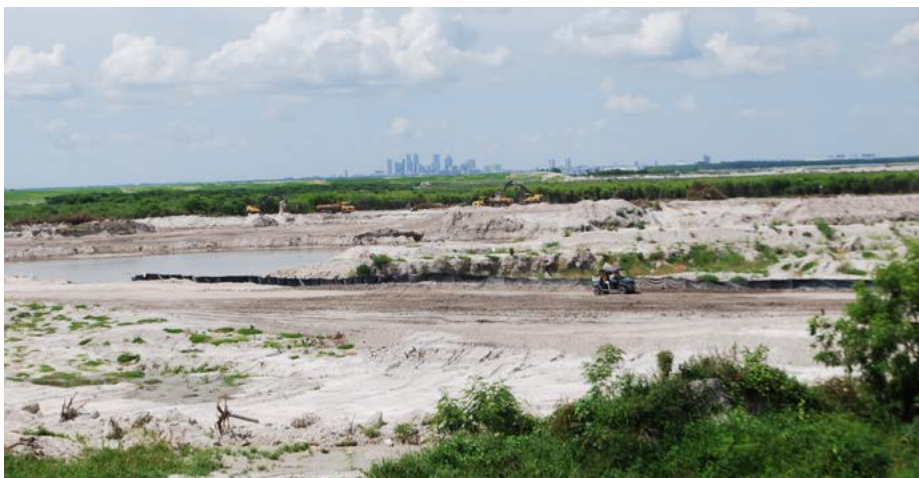
Two manmade islands in Tampa Bay are important disposal sites for dredged material. Photo courtesy Port Tampa Bay.
