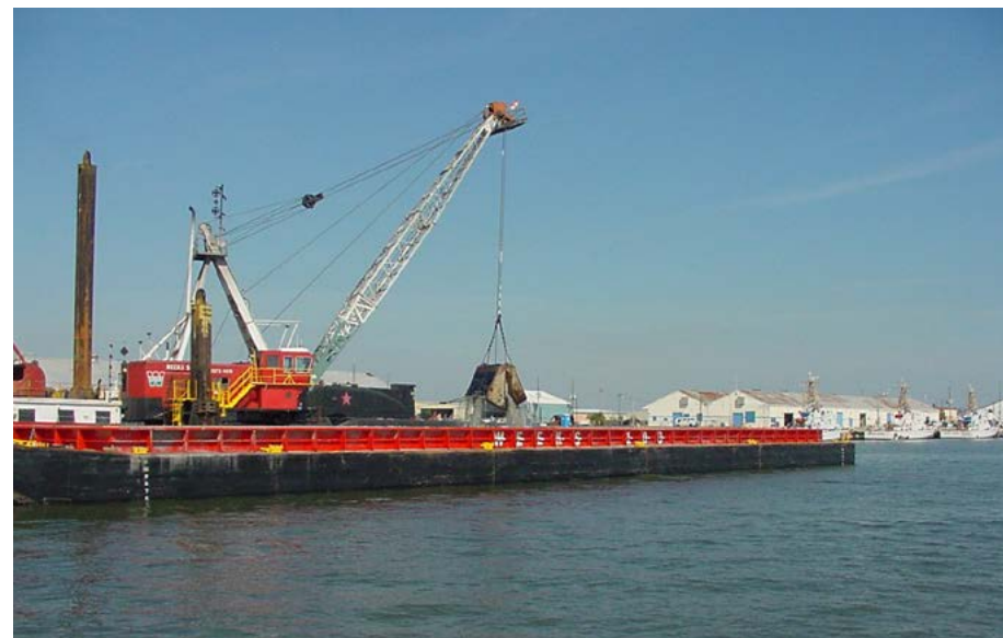
Clamshell dredging in Tampa Bay. This technique uses a “clamshell” bucket with hinged jaws, suspended from a crane aboard a barge. Photo by Nanette O’Hara.
