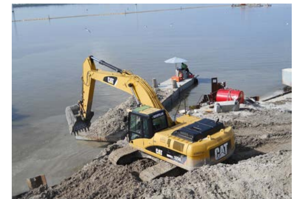
A deep dredge hole at Port Tampa Bay has been partially filled to improve water quality. Photo by Dennis Crnolatas.
